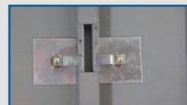
User doors reinforced at latches
