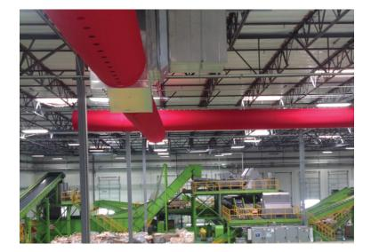
Technology advancements in fabric have created an opportunity for DuctSox to be used in applications where there are specific performance requirements. Anti-static fabrics are ideal for data centers and anti-microbial treated fabrics for laboratories, food processing and grow facilities.
